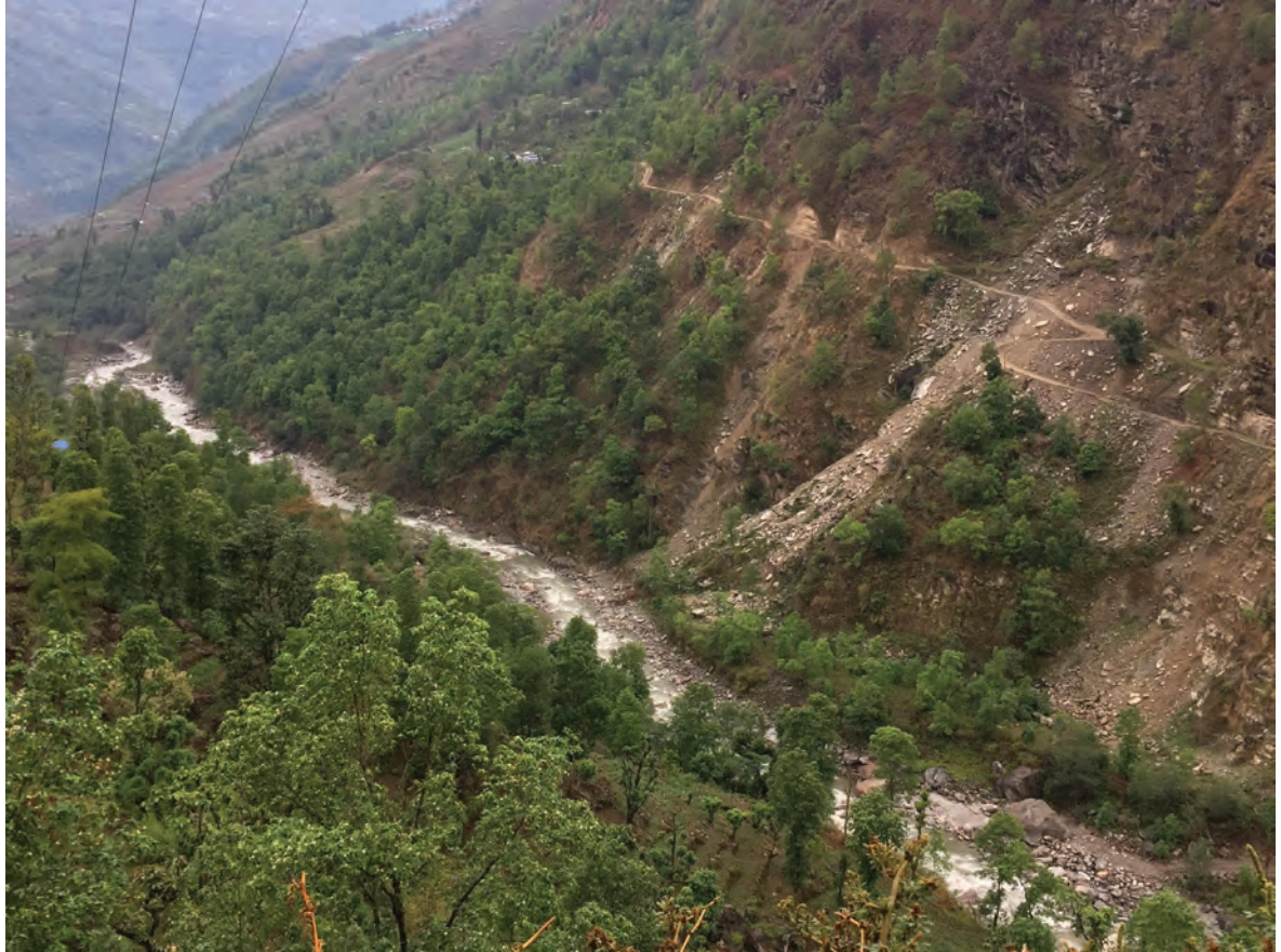
New roads constructed by Balephi Hydropower at the hillsides of Golche. Photo by Bina Limbu
