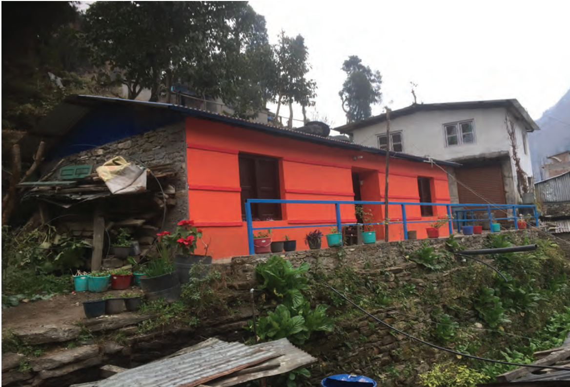
This two-roomed stone house was initially made up of two separate houses built by two separate grant beneficiaries belonging to the same family, and later, joined in the middle. Photo by Bina Limbu
