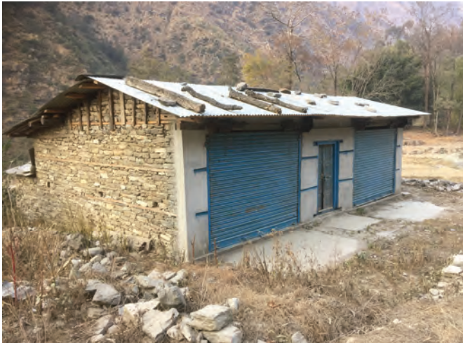
A non-compliant stone house at Manje built with two shutters at the front. Photo by Bina Limbu
